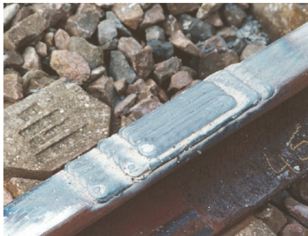
Figure 32. Area repaired by arc welding
