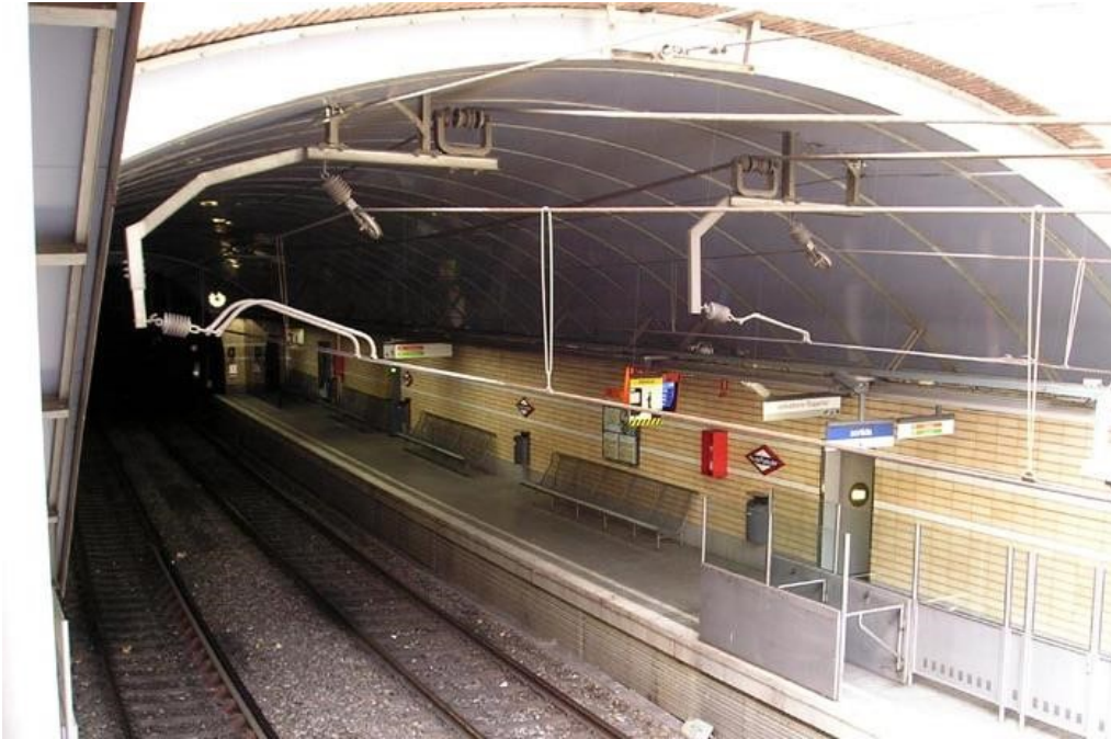
Figure 6. Overhead contact line in tunnel using cantilevers.
