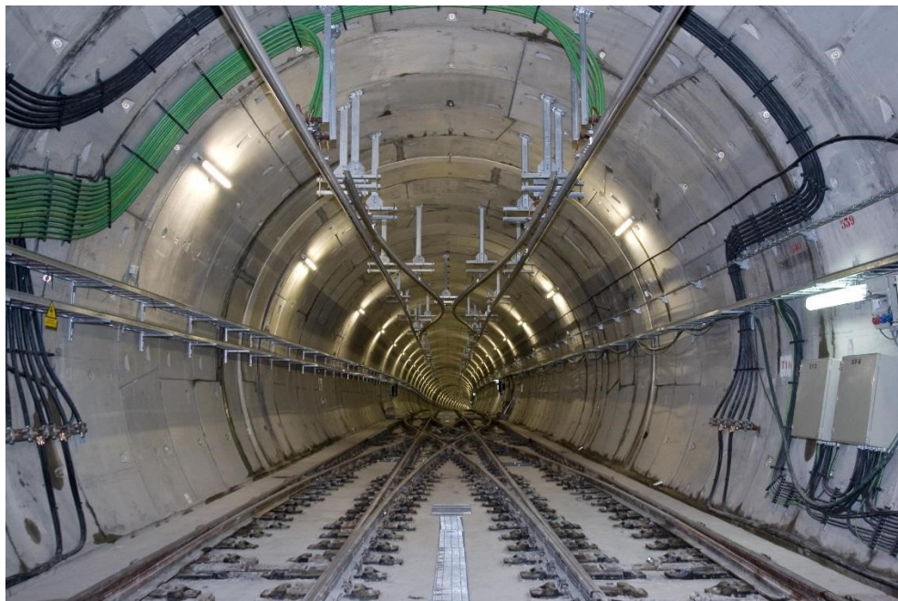
Figure 7. Rigid catenary in tunnel.
