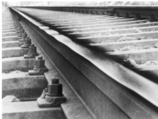
Figure 30. Corrugation wear
